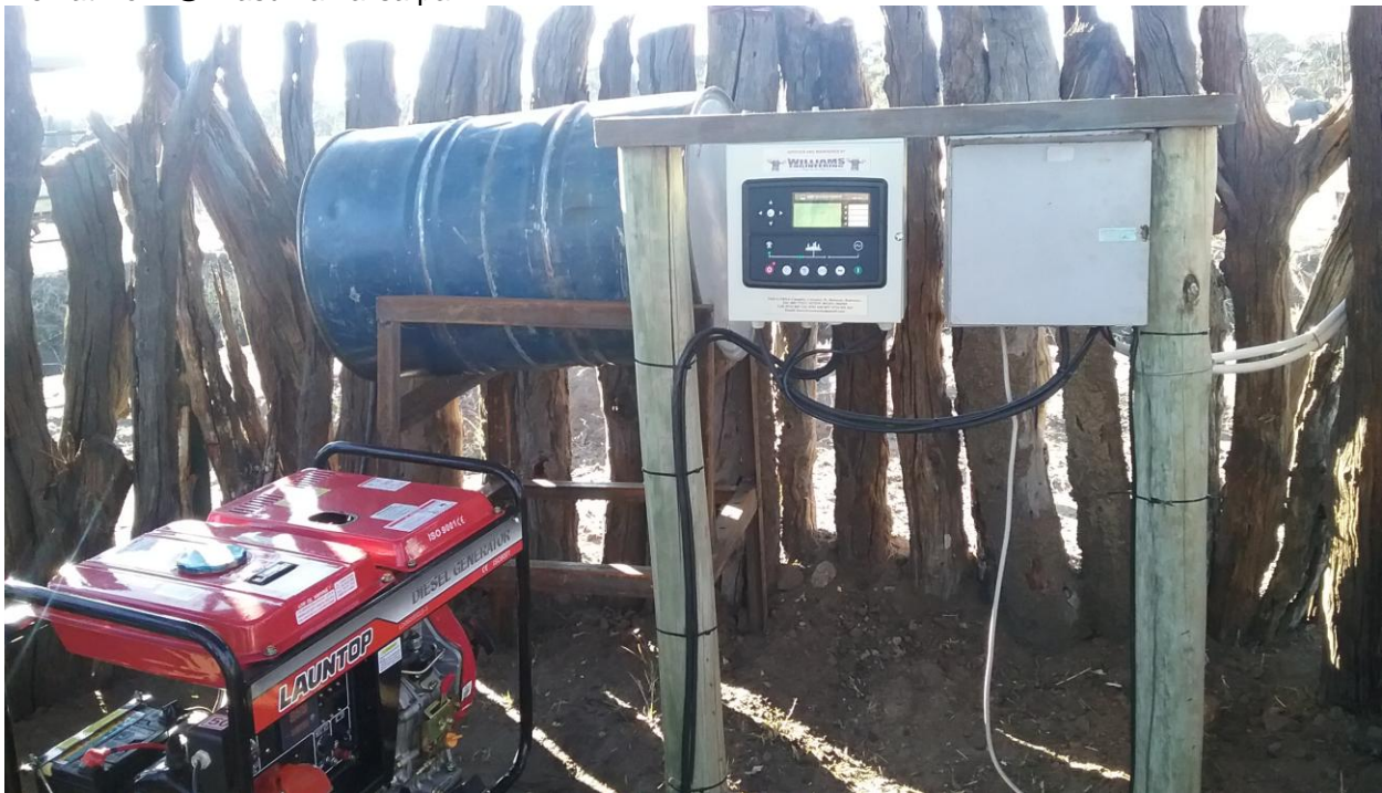
The newly purchased generators are automated and have been fitted and linked to the solar system which allows them to run automatically once the solar is turned off. It is timed to run during the night and it switches off during the day. This is currently installed at Chris' Pan.
