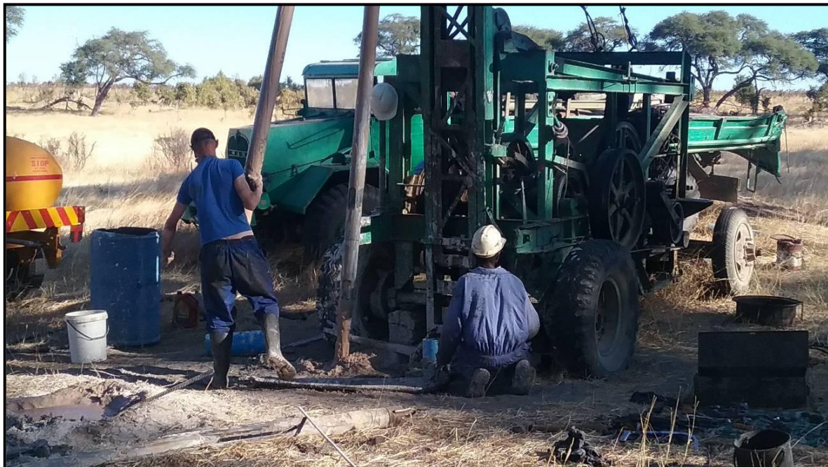
Pic 1. Work on the drilling of the Masomamalisa hole has started and is going on well. Now in order to drill in the sandy Kalahari soils, a special kind of drilling machinery and technology is needed so that there is very little disturbance to the soil structure and water supply capacity of the borehole.
