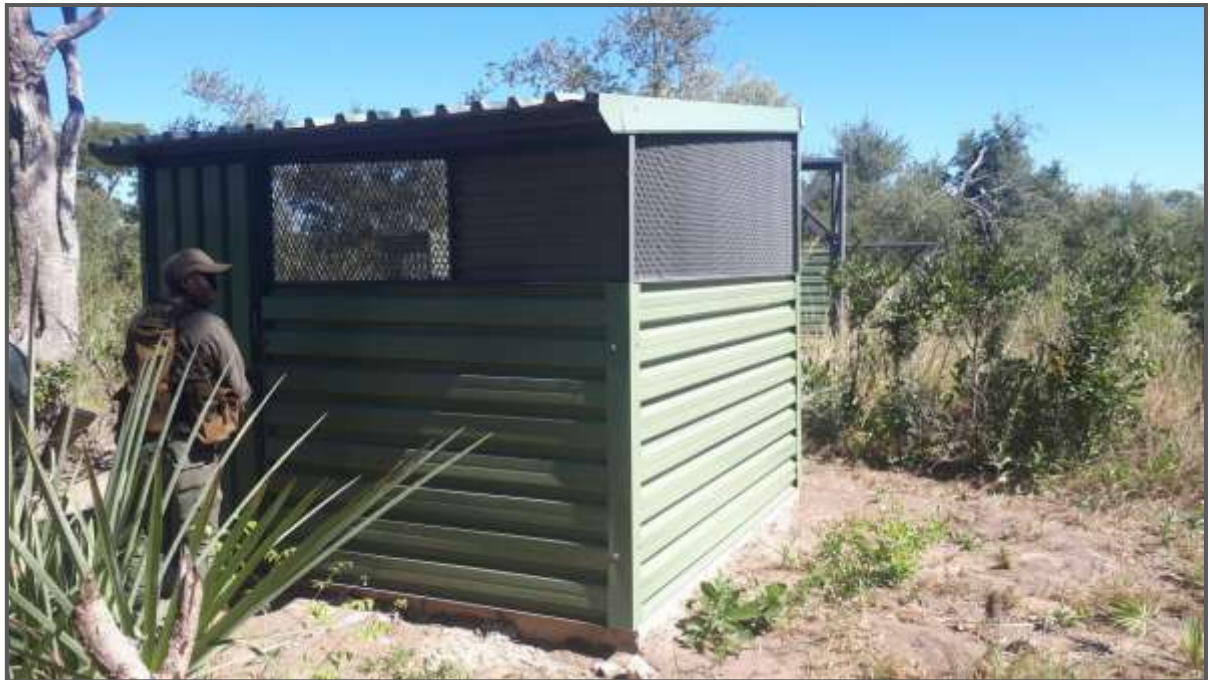
The barracks and kitchen at the new Bomani APU base
